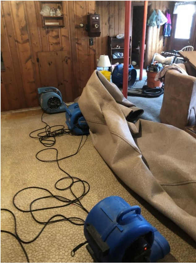
Equipment set up to dry wall to wall carpet on the same loss as the pictures prior to and below this one.
