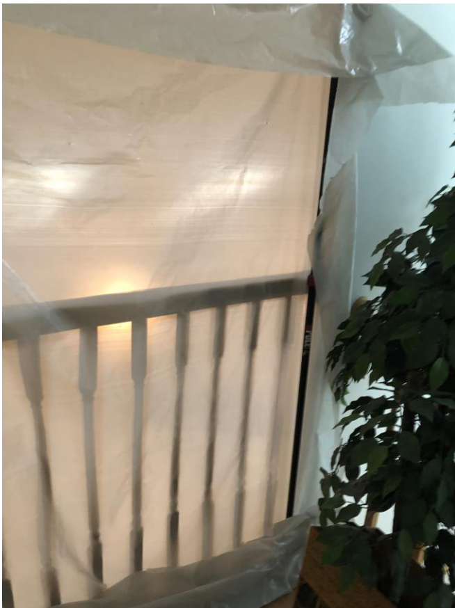
Containments – Second floor opera window opens to the Great Room. This is immediately adjacent to the Master Suite and bedroom two on the second floor.
