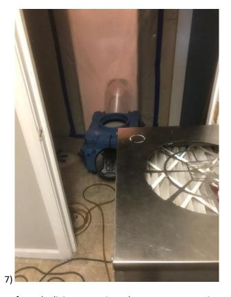
We used another containment "wall" at the bathroom door way from the living room since there were two entries to this bathroom/laundry combination. Layflat ducting attached to the air filtration device (AFD) by which clean filtered air is exhausted through a small slit cut into the plastic barrier. On a loss like this, all drying is done using the dehumidifier as the only drying equipment (no fans!!) thereby avoiding blowing around mold spores that were obviously present.
