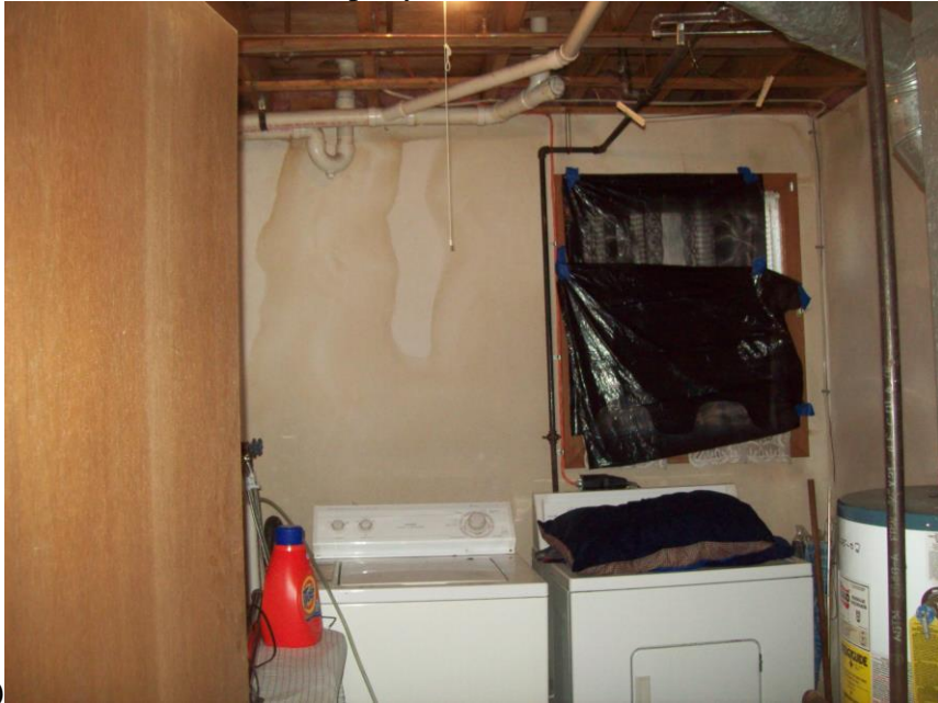
9) Basement laundry room
