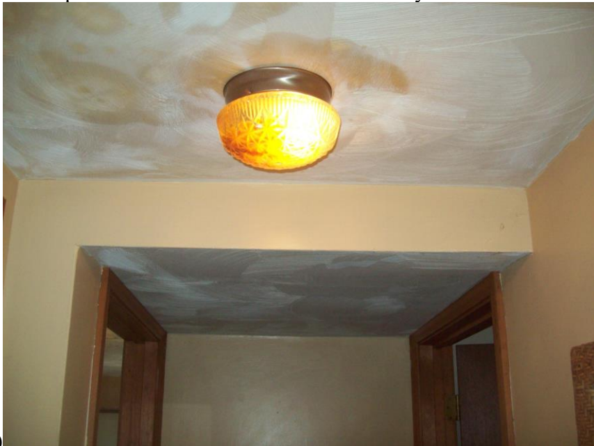
Lower level images - The entire globe of this light was filled with water and this is the ceiling in the family room.
