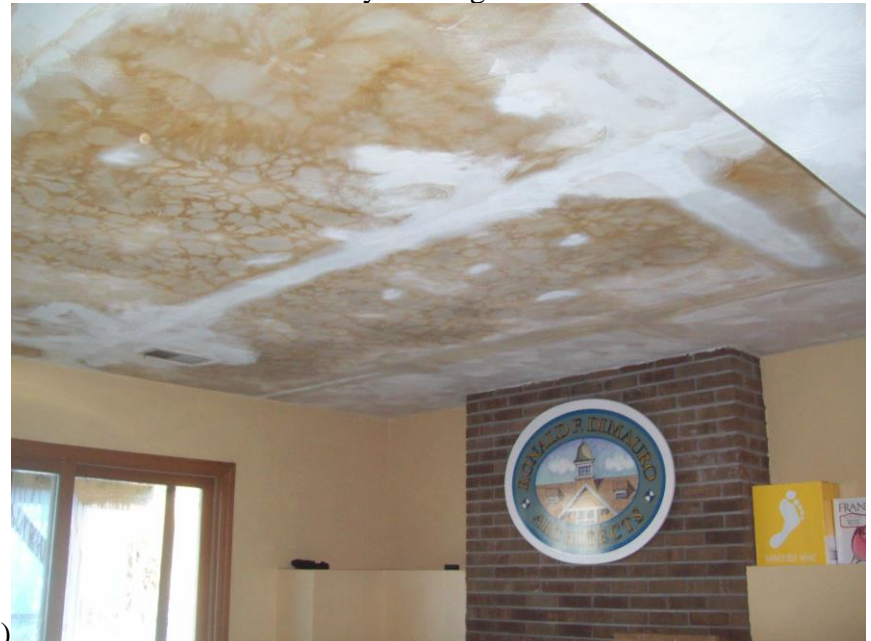
Lower level images - The entire globe of this light was filled with water and this is the ceiling in the family room.
