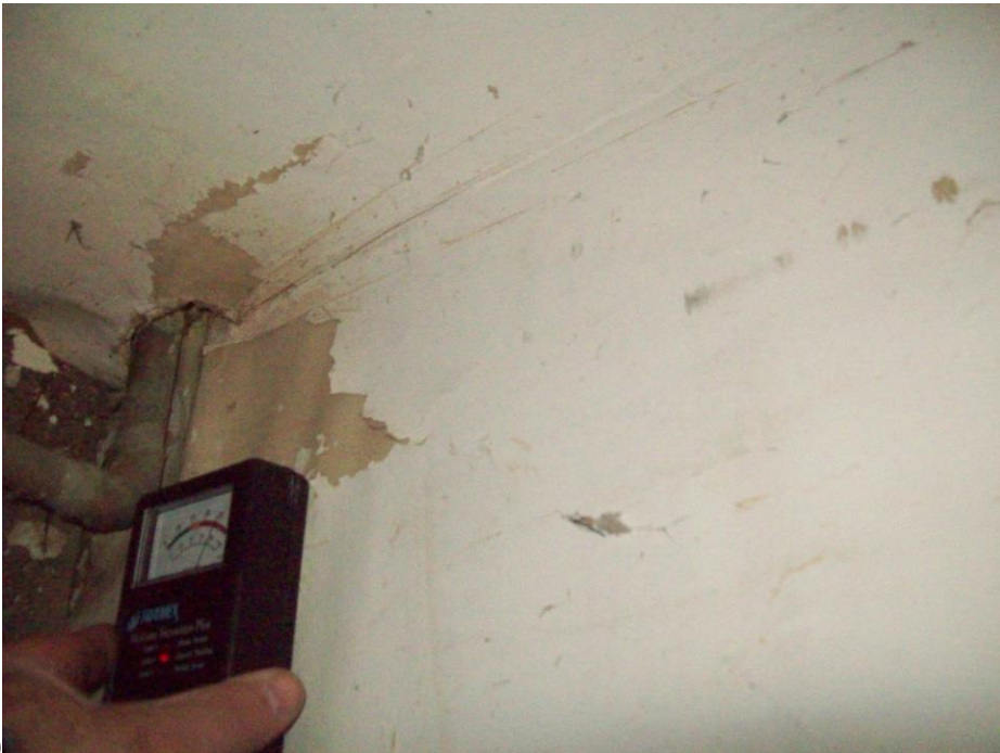
Wet exterior wall in the boiler alcove
