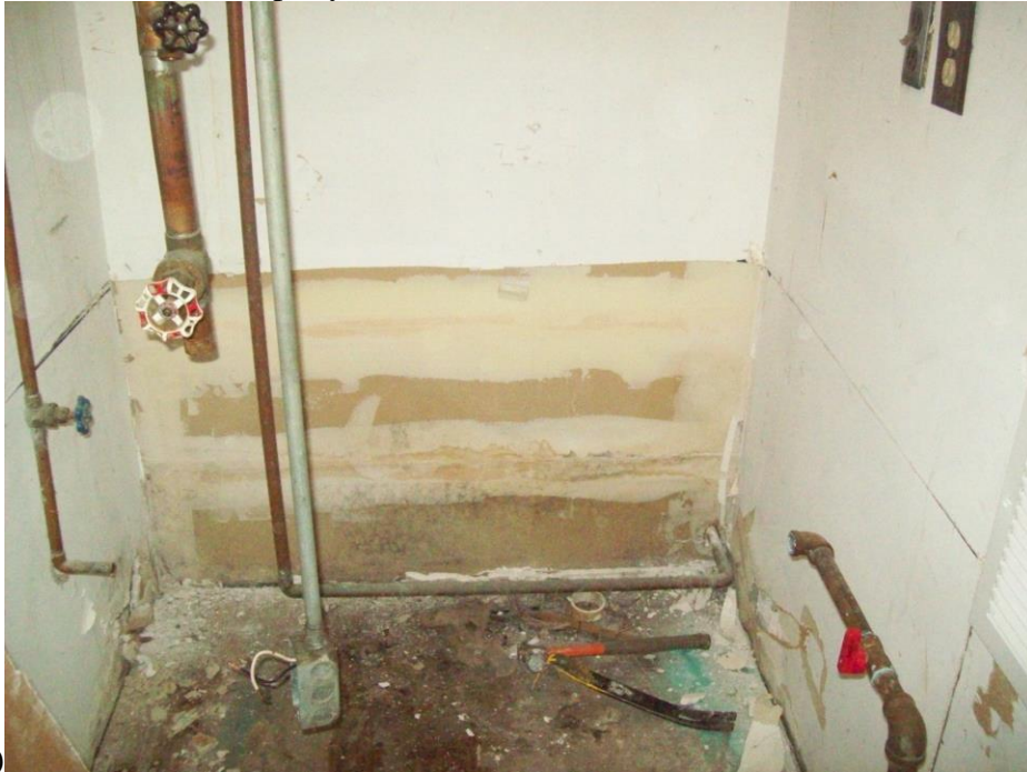
After mold confirmed, abatement started – double walled drywall
