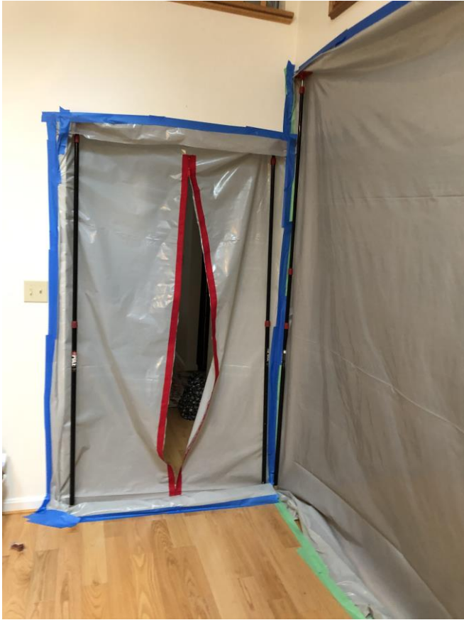
Containments set for mold abatement
