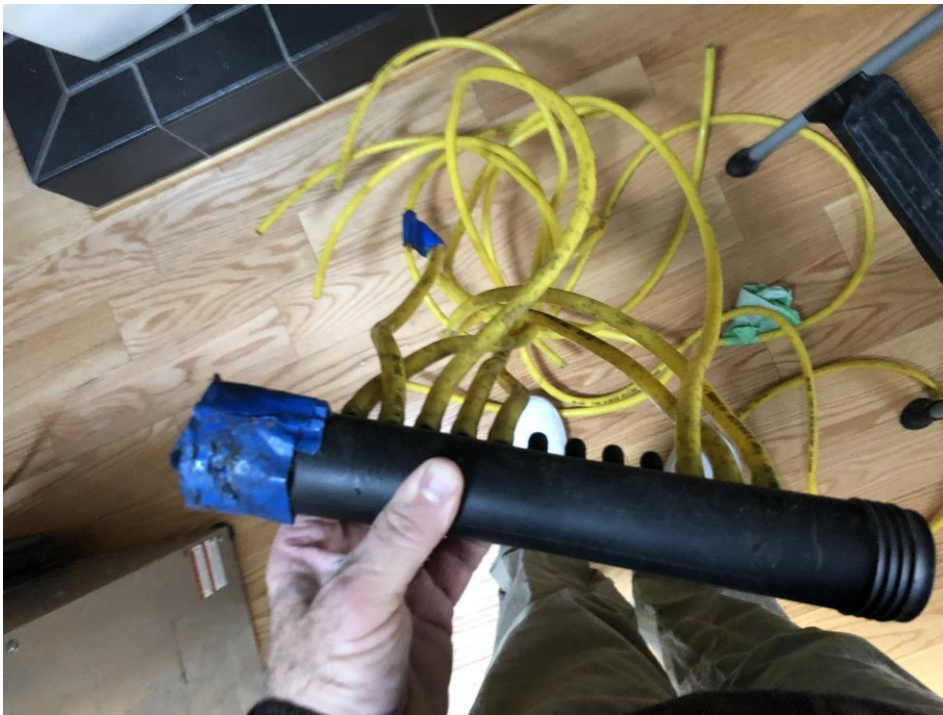
InterAir 1/2 Inch cavity feed was run into the ceiling
