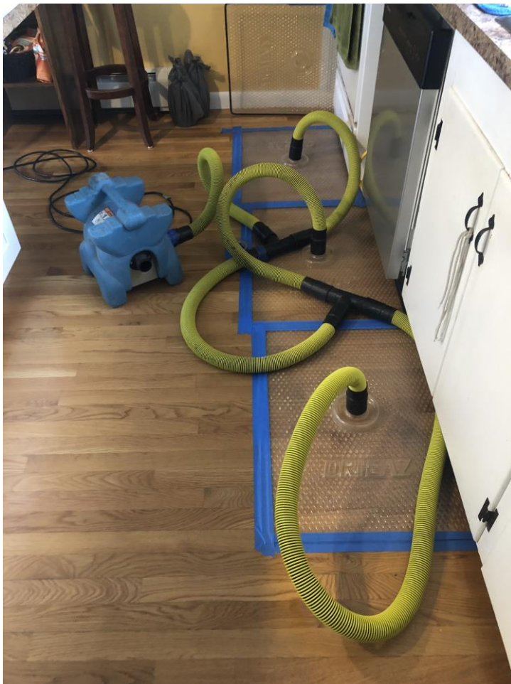
#12) Kitchen image at emergency response #13) Hardwood floor drying equipment 3/31/2022
