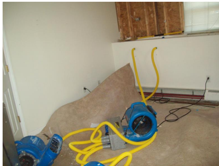
Basement wall and carpet dryout – We will not be able to save the carpet due to heavy saturation and stains previously mentioned.
