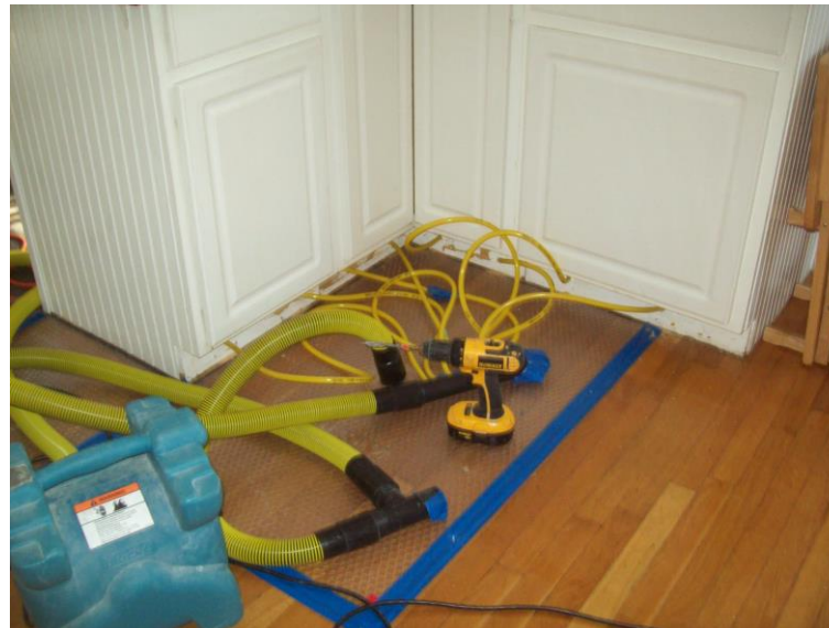
Rescue mat system using the DriEaz InterAir system blowing air in through the toe-kick to salvage cabinets
