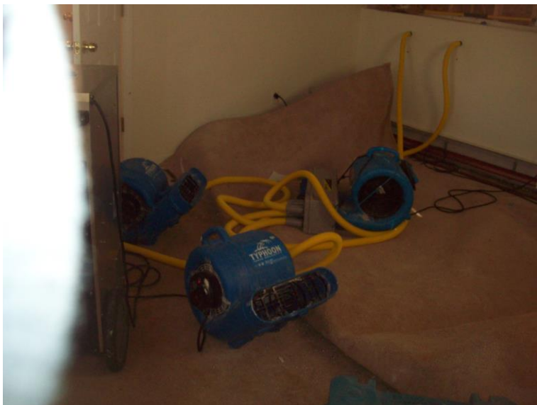
Basement wall and carpet dryout – We will not be able to save the carpet due to heavy saturation and stains previously mentioned.
