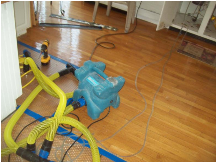
Rescue mat system using the DriEaz InterAir system blowing air in through the toe-kick to salvage cabinets
