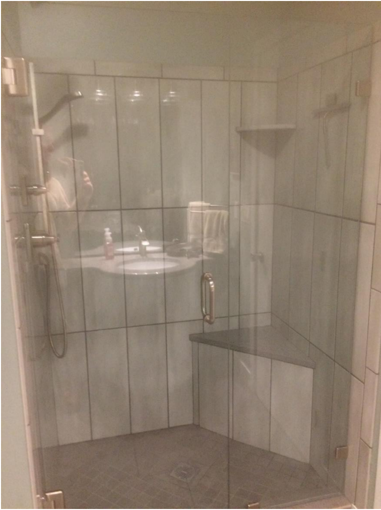
Glass door system was an in or out swing, with brushed nickel hardware
